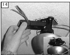
Install remote receiver by sliding into opening in the Mounting bracket. Make sure that the dip switches on the Transmitter and the Receiver are set to the same position. See Fig 32 for remote operation
